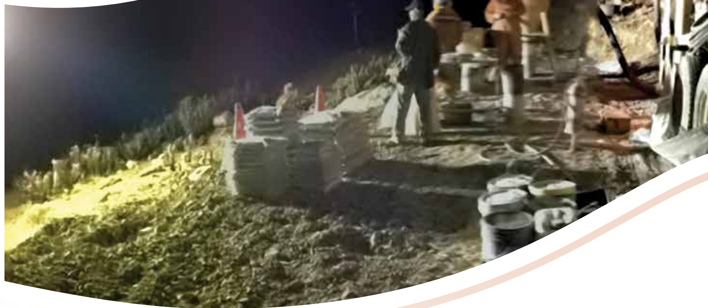
Night shift drilling at Soberana (July 2012)
