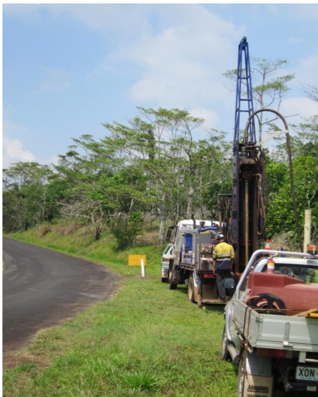
Figure 7 South Johnstone Drilling
