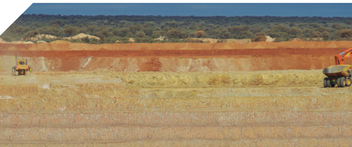
GARDEN WELL PIT
