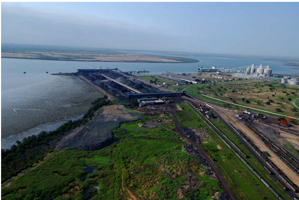
Diagram 3: Grindrod and Vitol's Matola Coal Terminal, Maputo. New coal stockpiles will be built to the left of this image on reclaimed land. Image by courtesy of Grindrod
