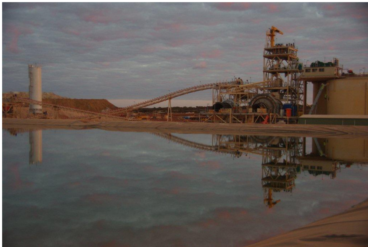
Processing plant at Garden Well
