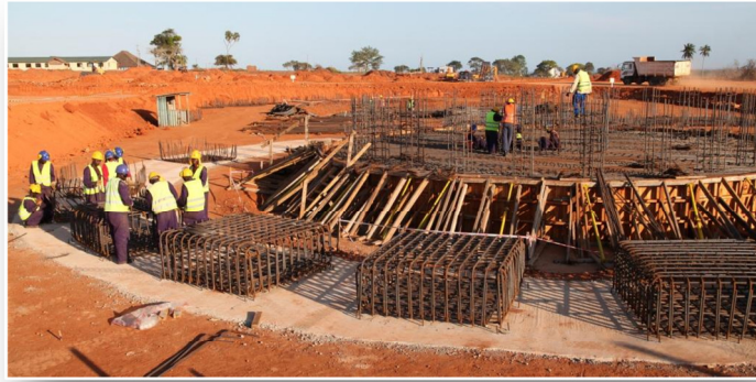
Form work for thickener foundation
