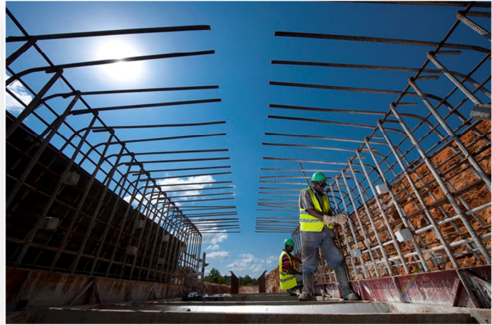
Diversion channel construction
