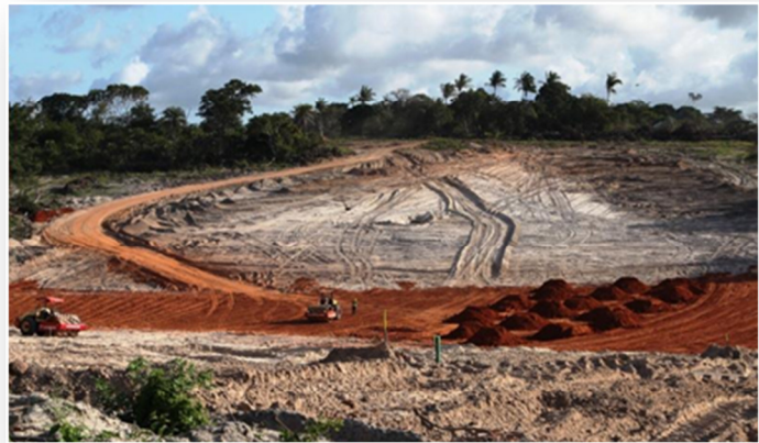
Tailings dam embankment foundations
