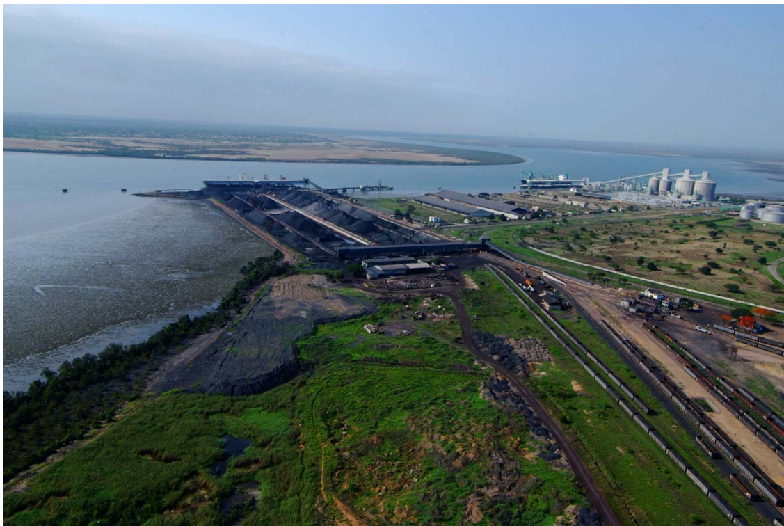
Grindrod and Vitol's Matola Coal Terminal, Maputo. New coal stockpiles will be built to the left of this image on reclaimed land. Image by courtesy of Grindrod
