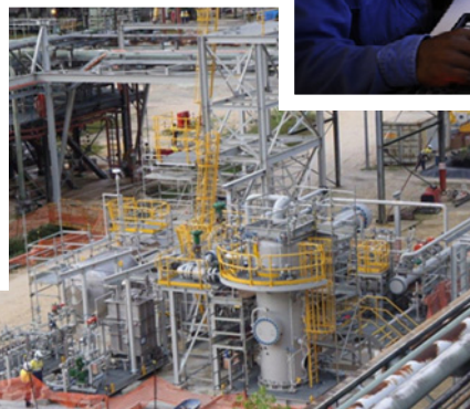
Commissioning Gas Unit - construction complete
