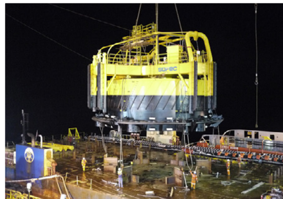
New CALM Buoy being lowered into position
