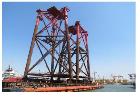
Wellhead platforms loadout from Tanggu yard
