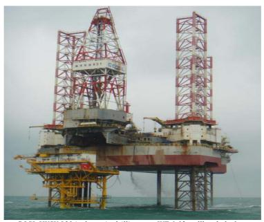
COSL HYSY 931 jack-up rig drilling over WZ 6-12 wellhead platform
