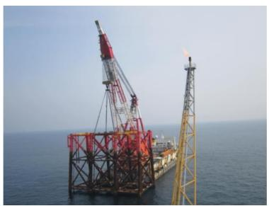
PUQB jacket lift by heavy lift vessel Lanjiang near CNOOC WZ 12-1 production complex
