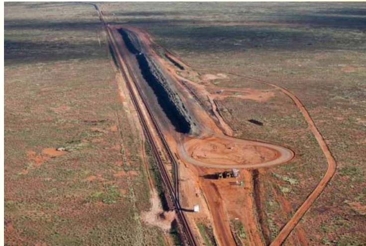
Rail Siding and Loading
