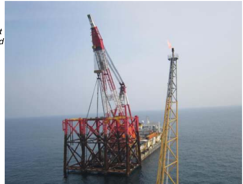
PUQB jacket lift by heavy lift vessel Lanjiang (Right)
