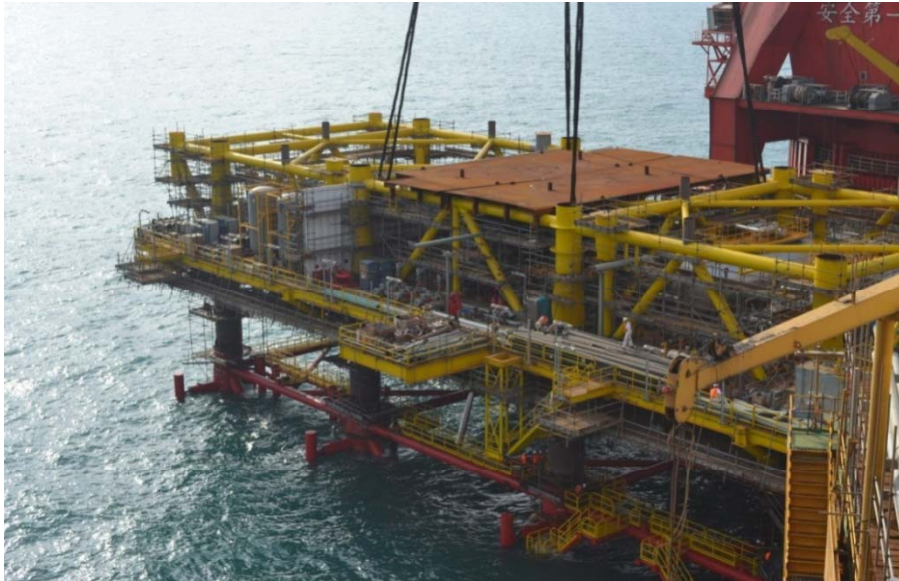
PUQB module support frame being lifted onto platform jacket
