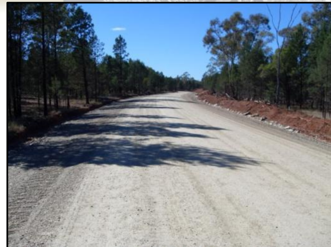
All weather access road complete
