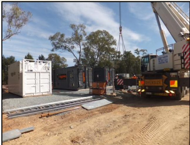
Decline power station installed
