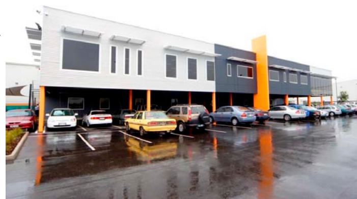
10 Butler Boulevard, Adelaide Airport, SA
