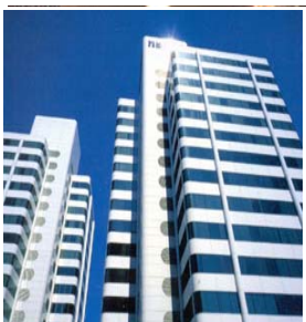
Chatswood Towers, NSW
