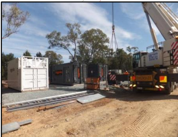
Installing Decline Power Station
