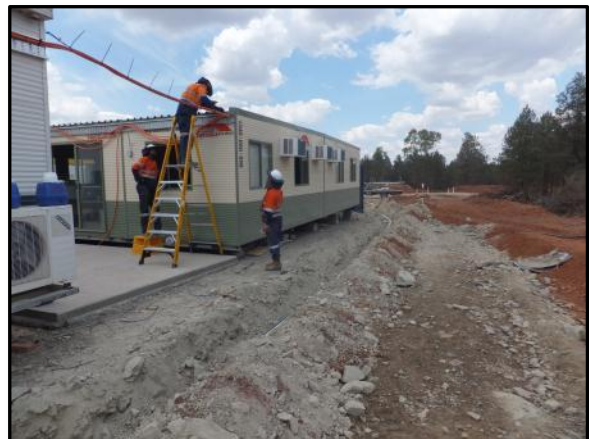
Pybar Office Installation
