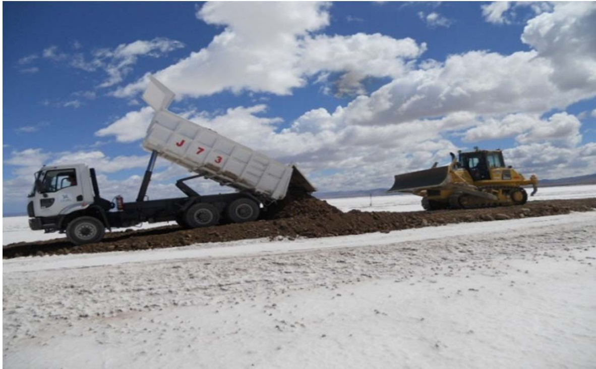
Figure 1 Building Road to Bore Field
