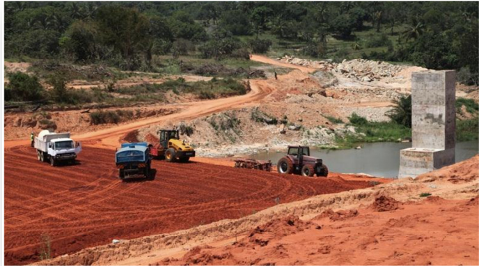
Dam coffer wall construction
