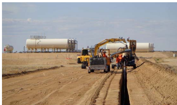
Bauer to Lycium pipeline installations – PEL 91
