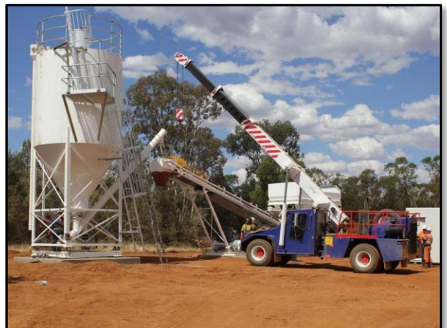
Installation of concrete batch plant
