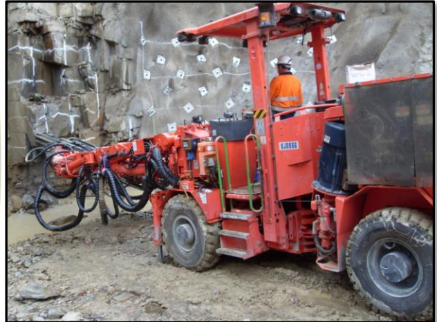
Jumbo boring first portal cut
