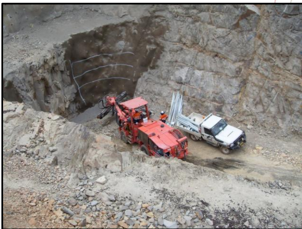
Jumbo preparing for first portal cut
