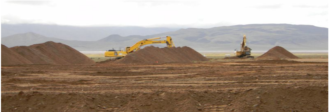
Figure 8: Construction of Evaporation ponds
