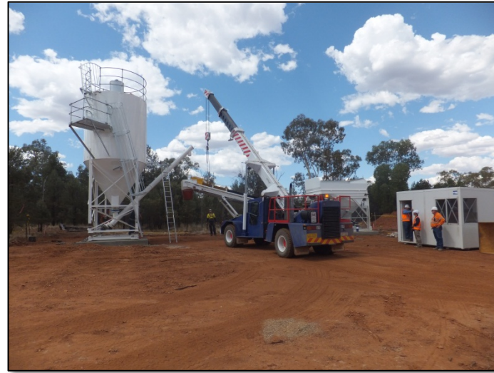
Batch plant installation
