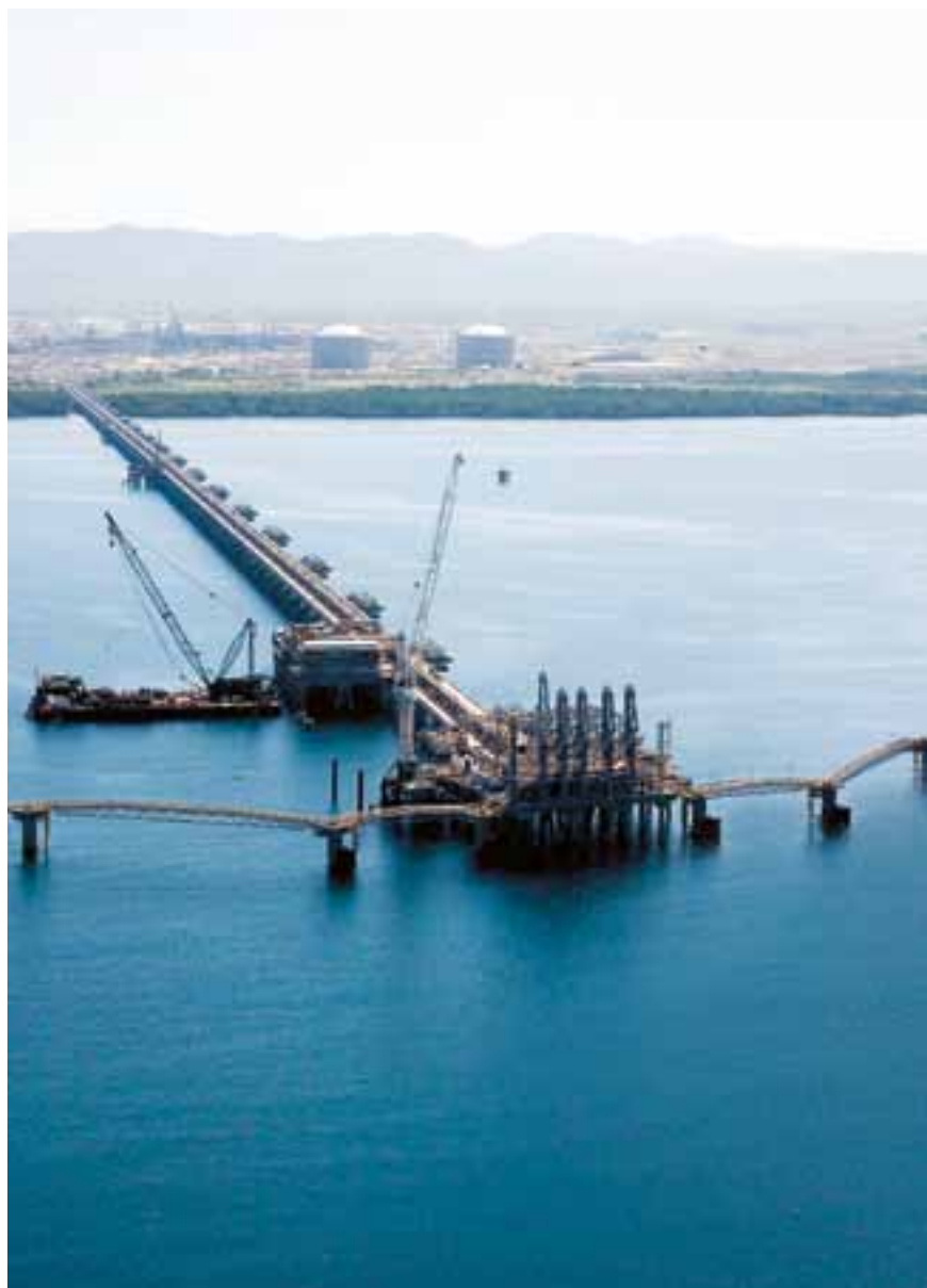
PNG LNG Project export jetty located outside Port Moresby, PNG
