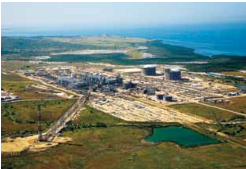
PNG LNG Project Plant site, near Port Moresby, PNG
