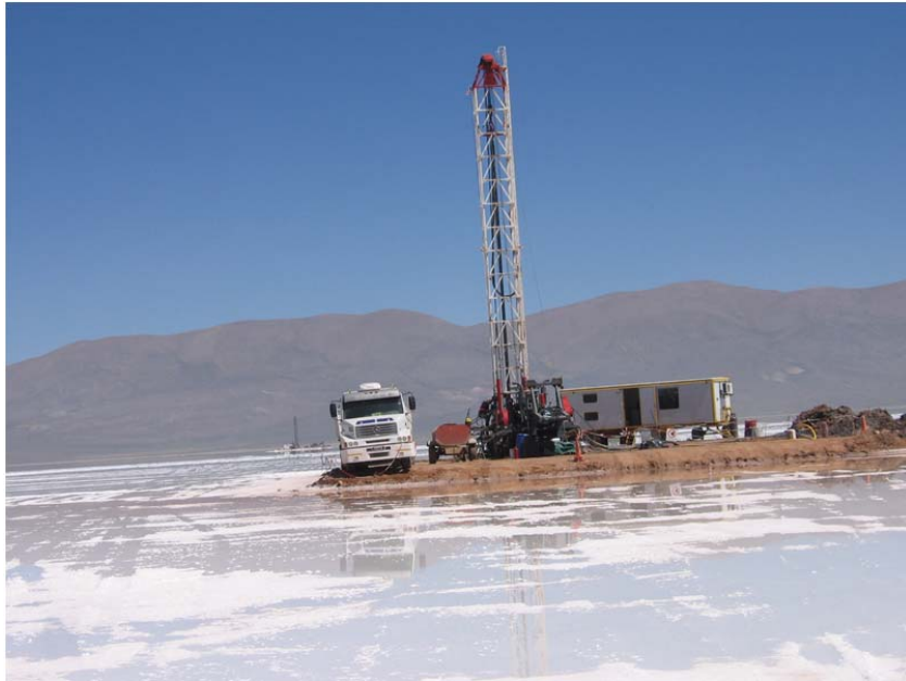
Drilling bore holes for brine wells on the salar
