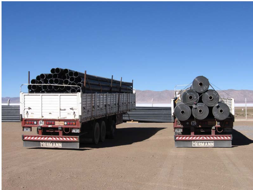
Pipes and liners for the evaporation ponds
