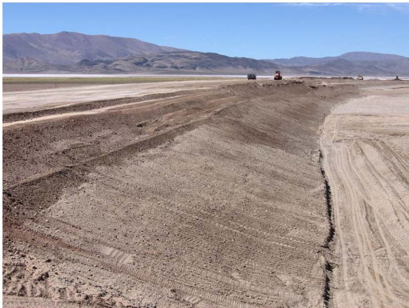
Internal road next to an evaporation pond under construction
