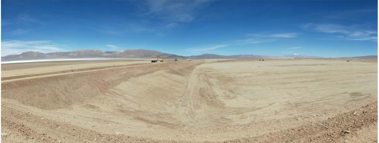
Evaporation pond nearing construction completion. The next step is to install the liner.
