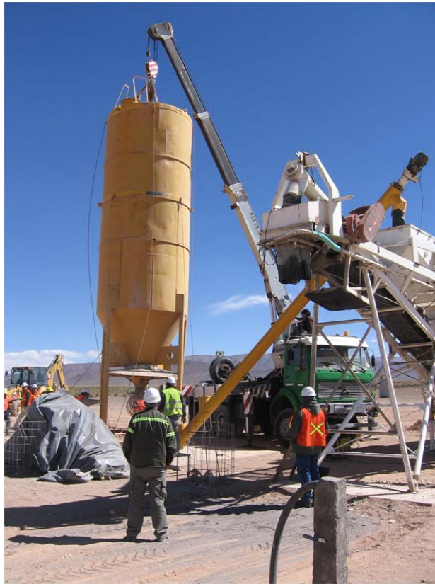
Silo installation for the effluent plant
