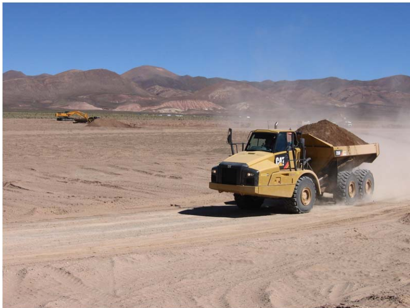
Making progress, on time and within budget
