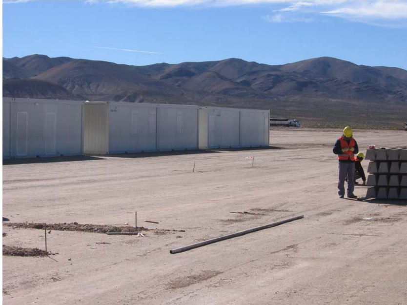
Camp accommodation under construction
