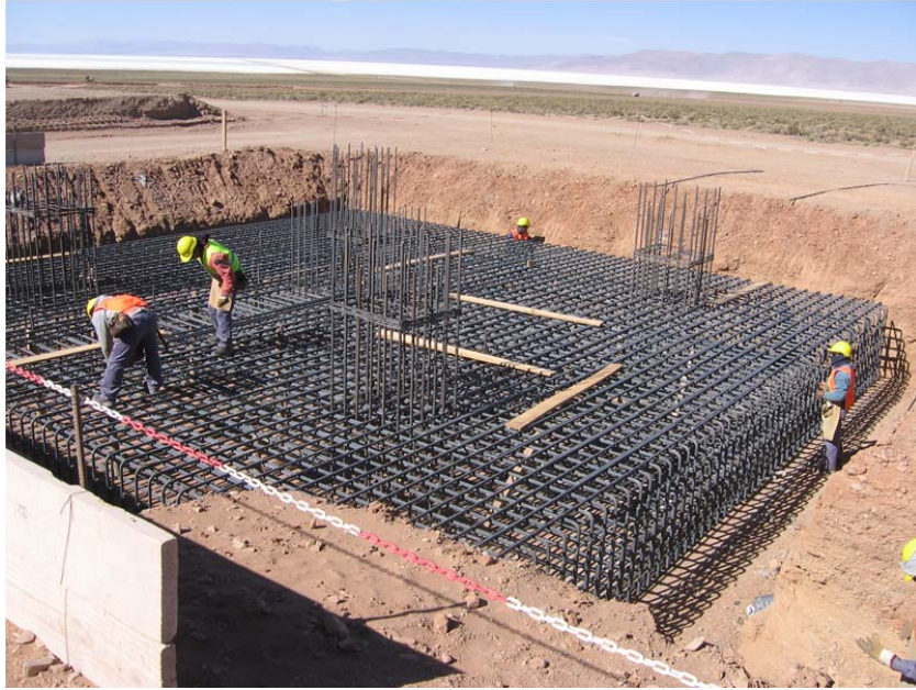
Liming Plant Foundations
