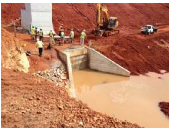
Culvert with plug in place
