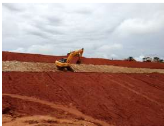
Armouring of dam wall
