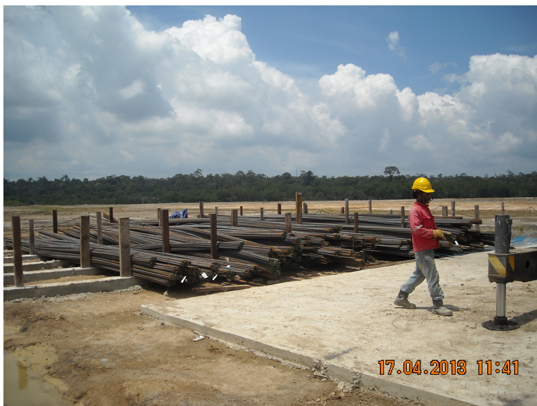
Reinforcing Bars for RC Foundation Works
