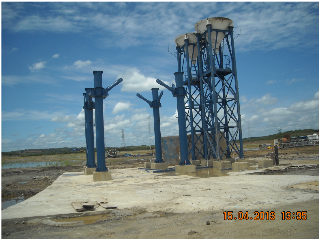
Steel Structures for Concrete Batching Plant
