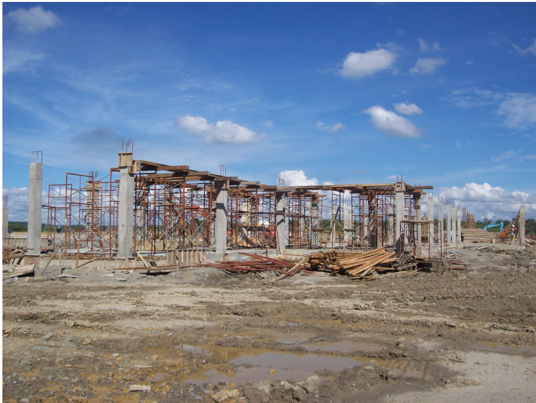
Construction of Control Building for Power Sub-Station
