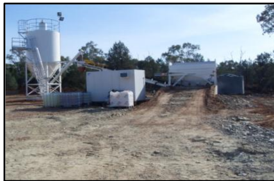
Completed concrete batch plant
