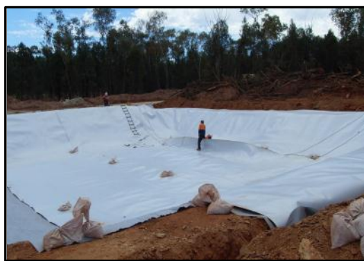
Installation of lined leachate ponds for the ROM pad
