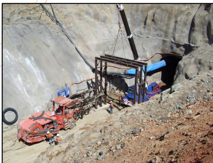
Installation of Vent Fan: Hera Project Portal
