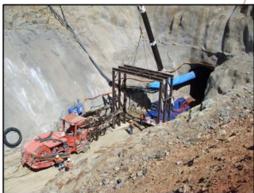
Installing Main Vent Fan at Portal face
