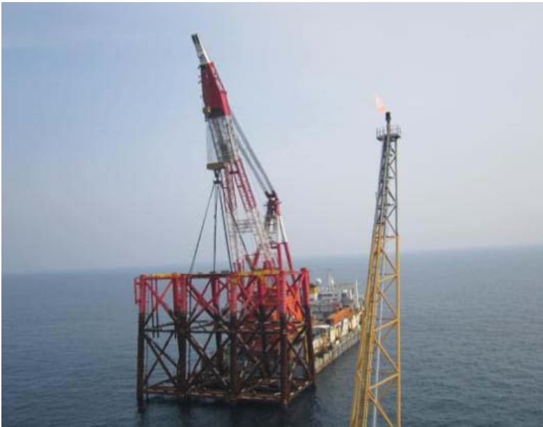
PUQB jacket lift by heavy lift vessel Lanjiang (L)
