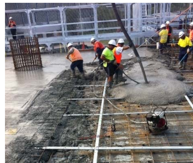
Field trials of ENVISIA TM concrete for the Barangaroo Project
