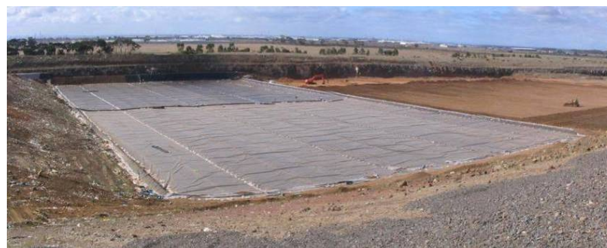
Deer Park landfill – New composite lined cell
