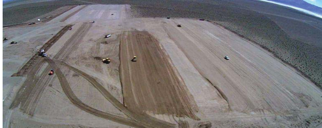
Aerial view of camp pad construction
