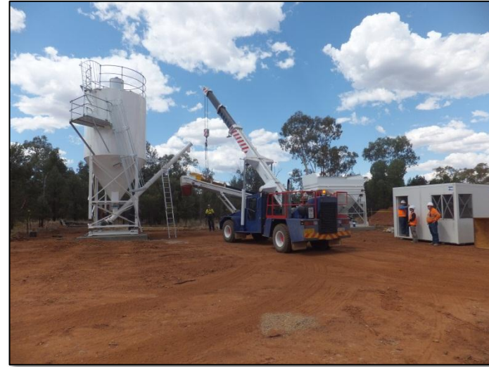
Batch plant installation
