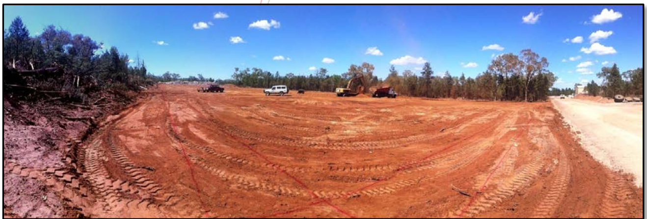
Clearing of ROM Pad area
