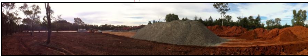
Clearing of process plant area
