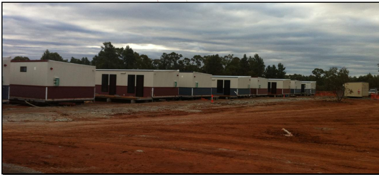
Accommodation units installed at Hera
