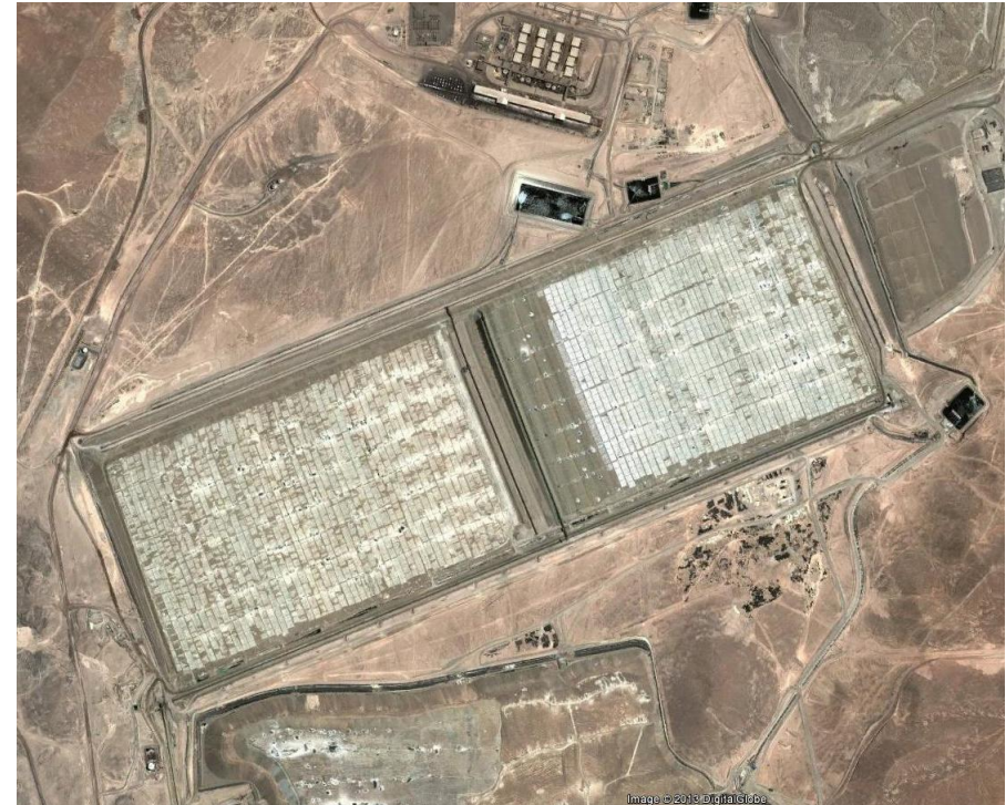
Barrick's Zaldivar Project leach pads, Chile
