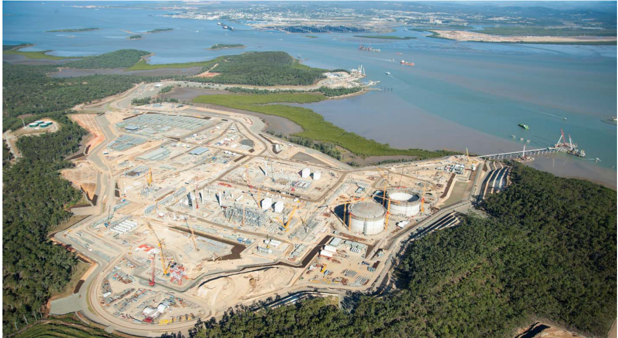
LNG plant site on Curtis Island, June 2013.
