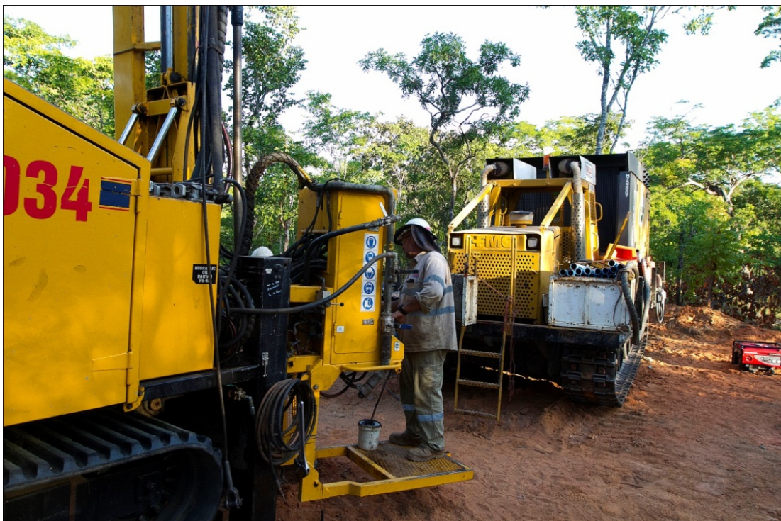
Figure 2: Drill Rig and Support Vehicle
