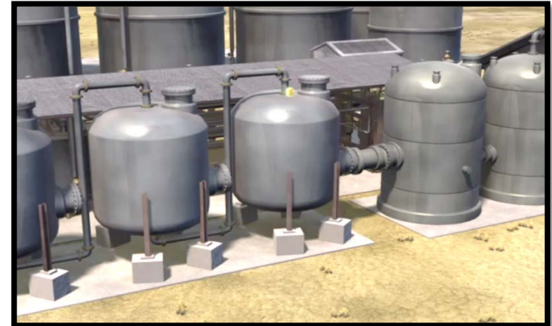
Central Processing Plant: Ion Exchange Vessels (left), Elution circuit (right)
