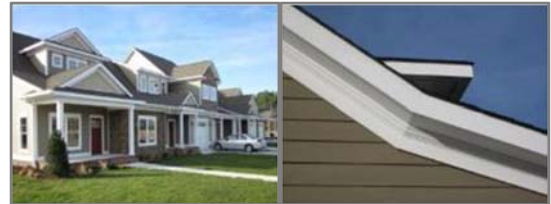
Multi Family New Construction – Gloucester, VA
