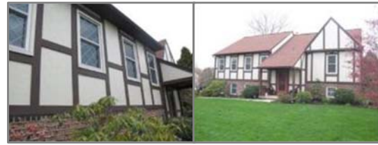
Repair & Remodel – Lancaster, PA
