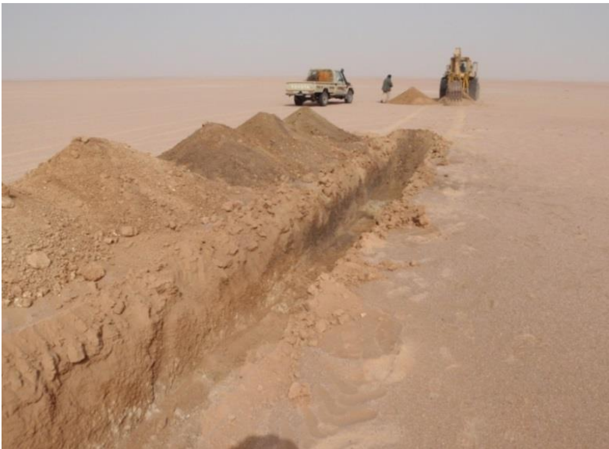
Trenching through the Reguibat calcretes showing the ease of excavation, and the flat, vegetation-free landscape
