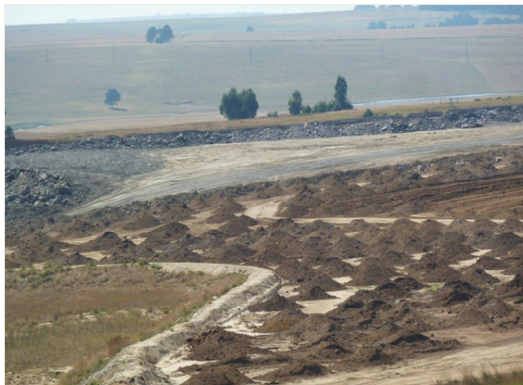
Topsoil being replaced after roll-over mining at the Ferreira North Pit
