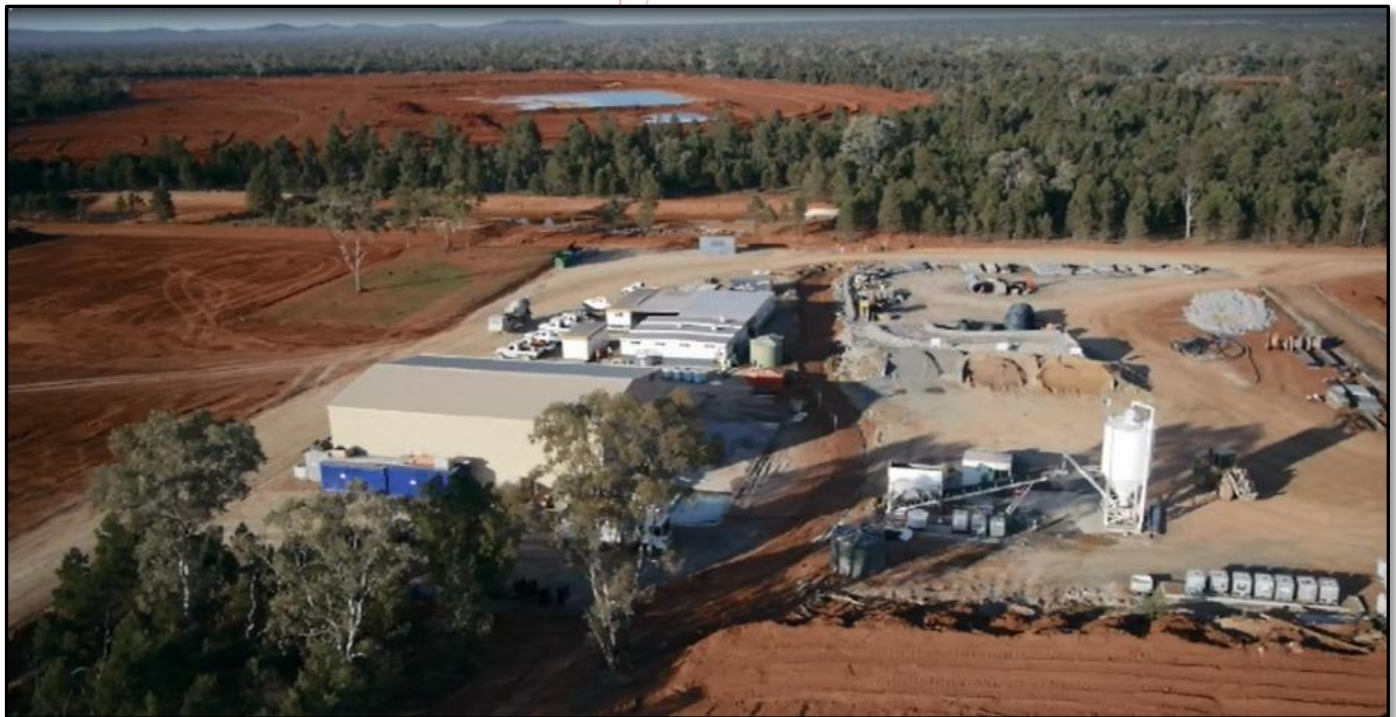
Contractors area, looking south with TSF construction in background
