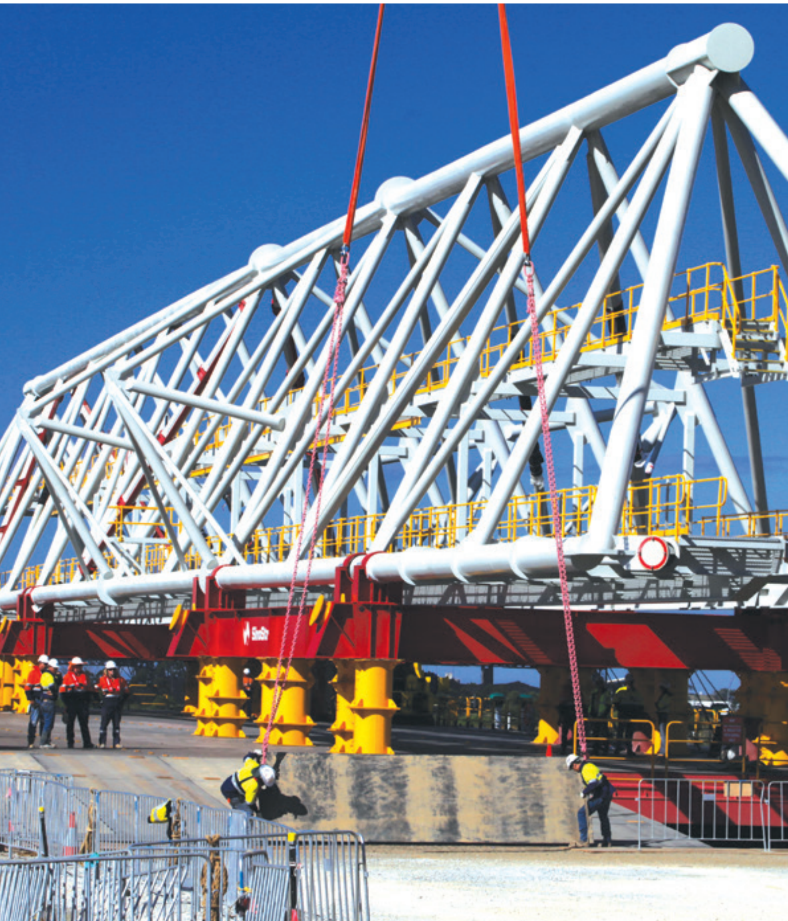
Monadelphous employees delivering a stacker bridge to Wiggins Island Coal Export Terminal, Gladstone, Queensland. At 15 metres wide, 125 metres long and weighing 377 tonnes this is the largest item built and shipped from China by Monadelphous's subsidiary, SinoStruct.
