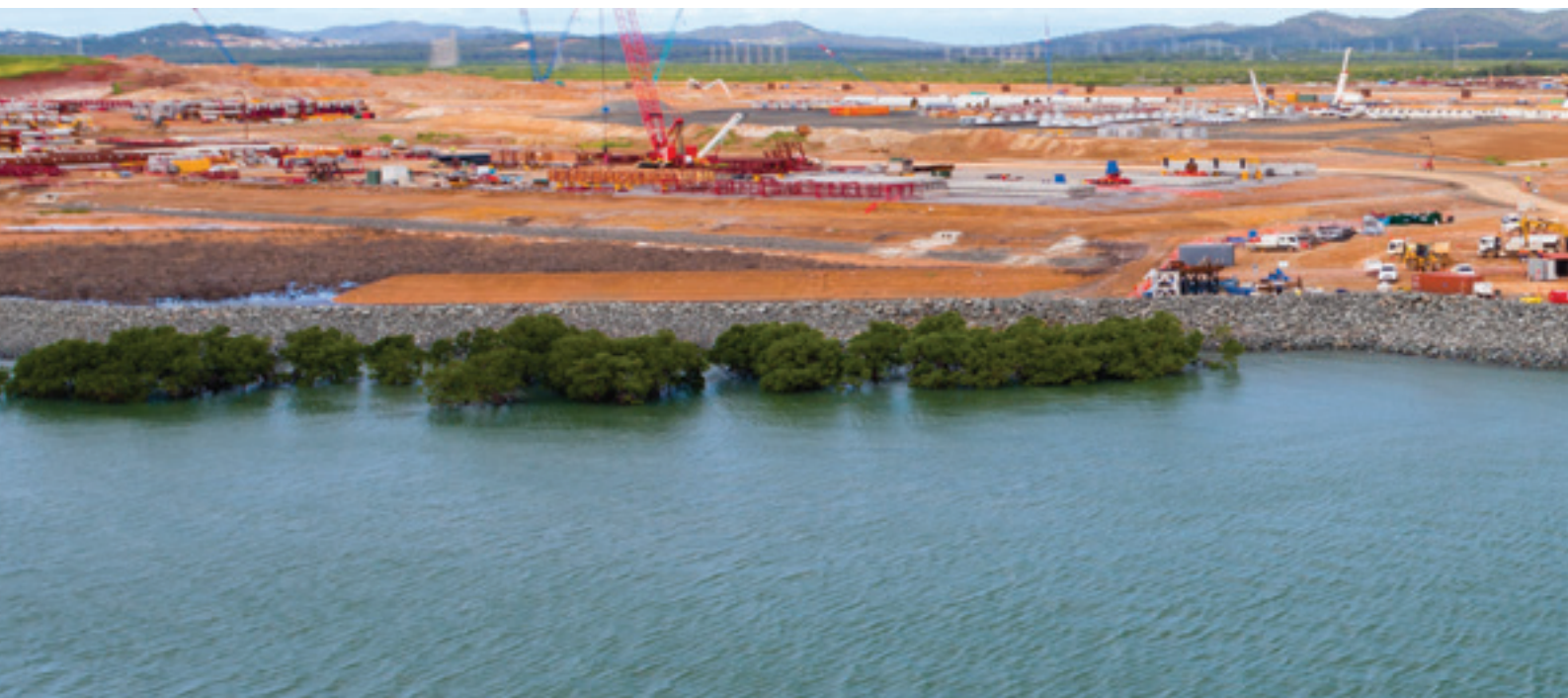
The purpose-built canti-traveller in operation at the Wiggins Island Coal Export Terminal wharf approach jetty built by Monadelphous Muhibbah Marine, Gladstone, Queensland. A canti-traveller is a purpose-built structure that installs piles into the seabed using an 'over-the-top' construction method.
