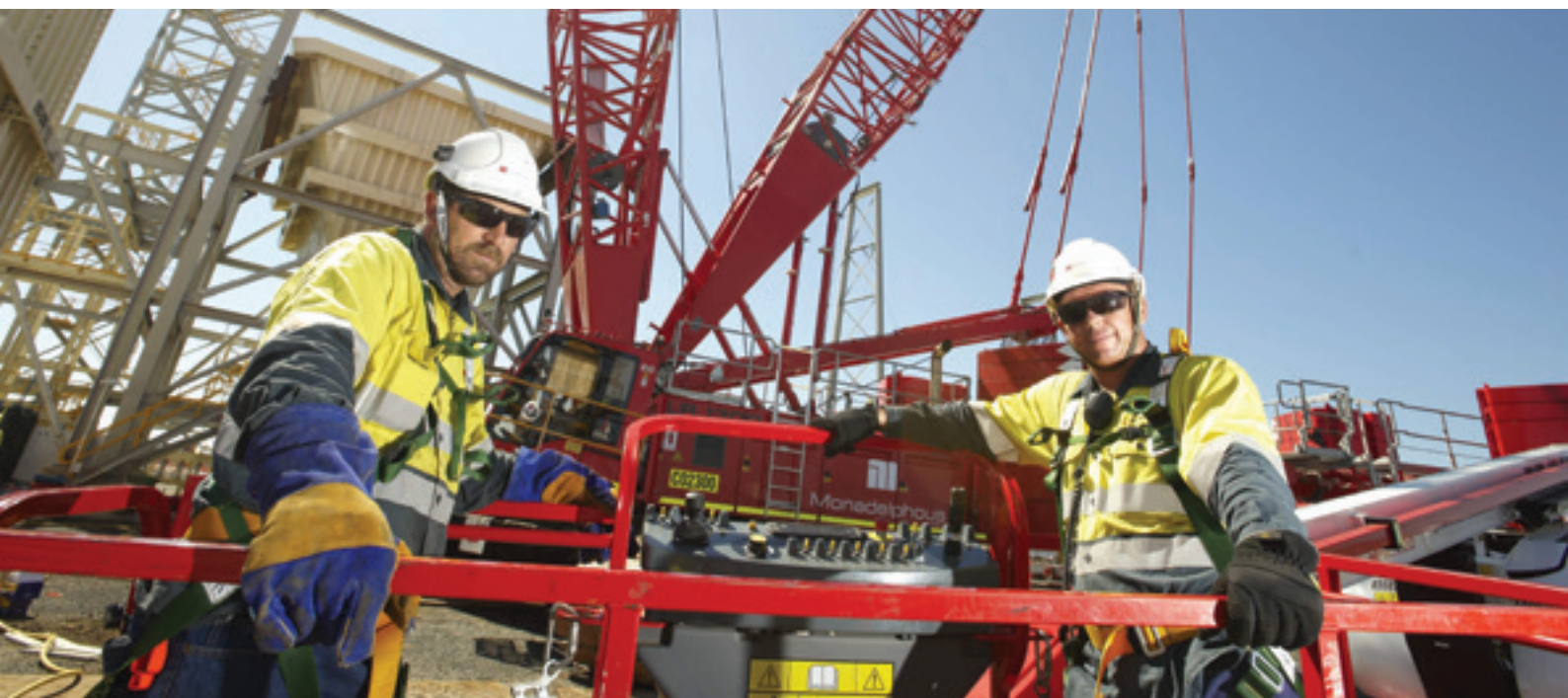
Monadelphous employees assembling the top section of the drift surge bin at a coal operation in Queensland.
