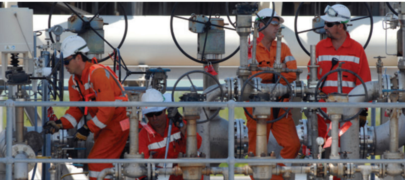
Mechanical crew perform maintenance duties at a shutdown at a LNG plant, Darwin, Northern Territory.
