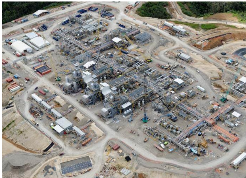
Hides Gas Conditioning Plant September 2013
