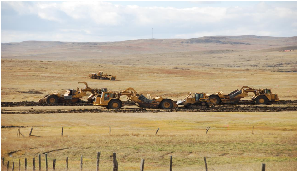
Figure 1: Earthworks commence at Peninsula's Ross Project Area, Wyoming USA
