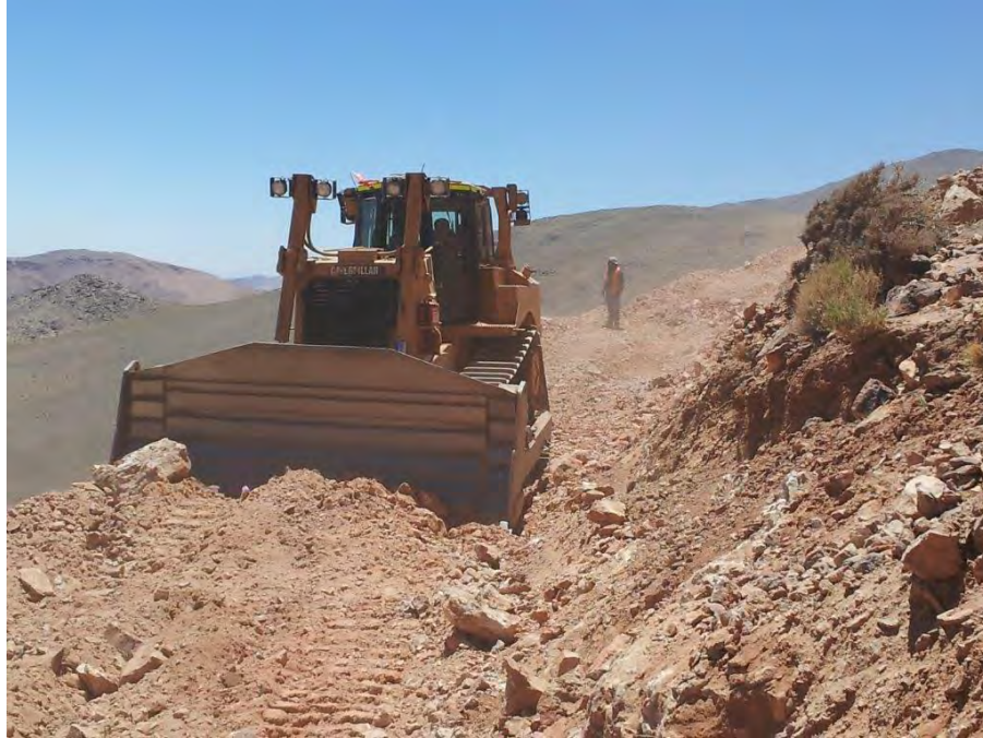
D8 engaged in track construction between pads, dozing in argillic altered porphyry. Red and yellow colours due to iron oxides and jarosite after pyrite.
