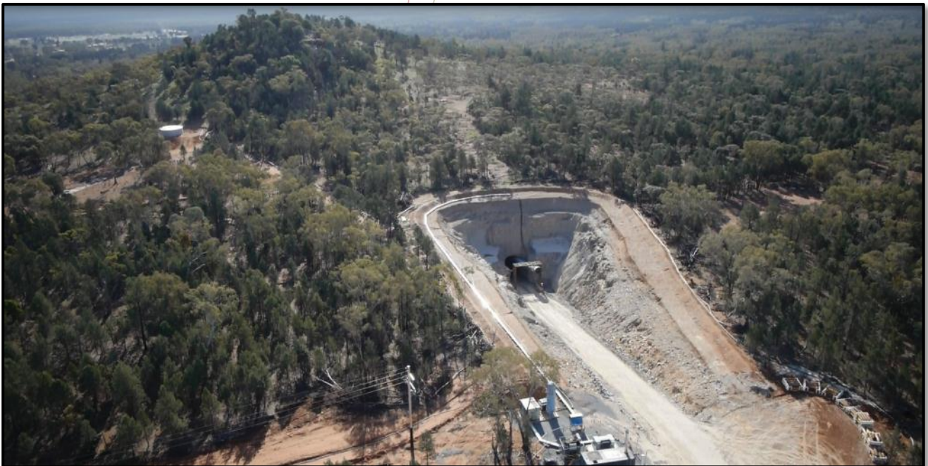
Hera Boxcut and Portal
