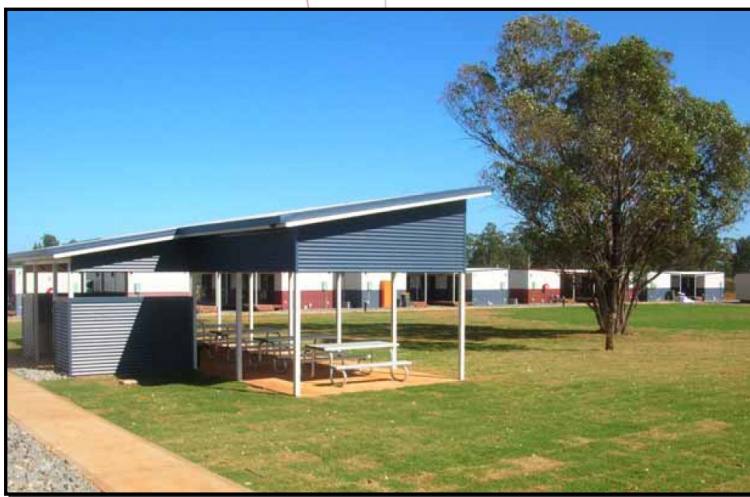
Hera Accommodation Camp – BBQ Area and Stage 1 accommodation units
