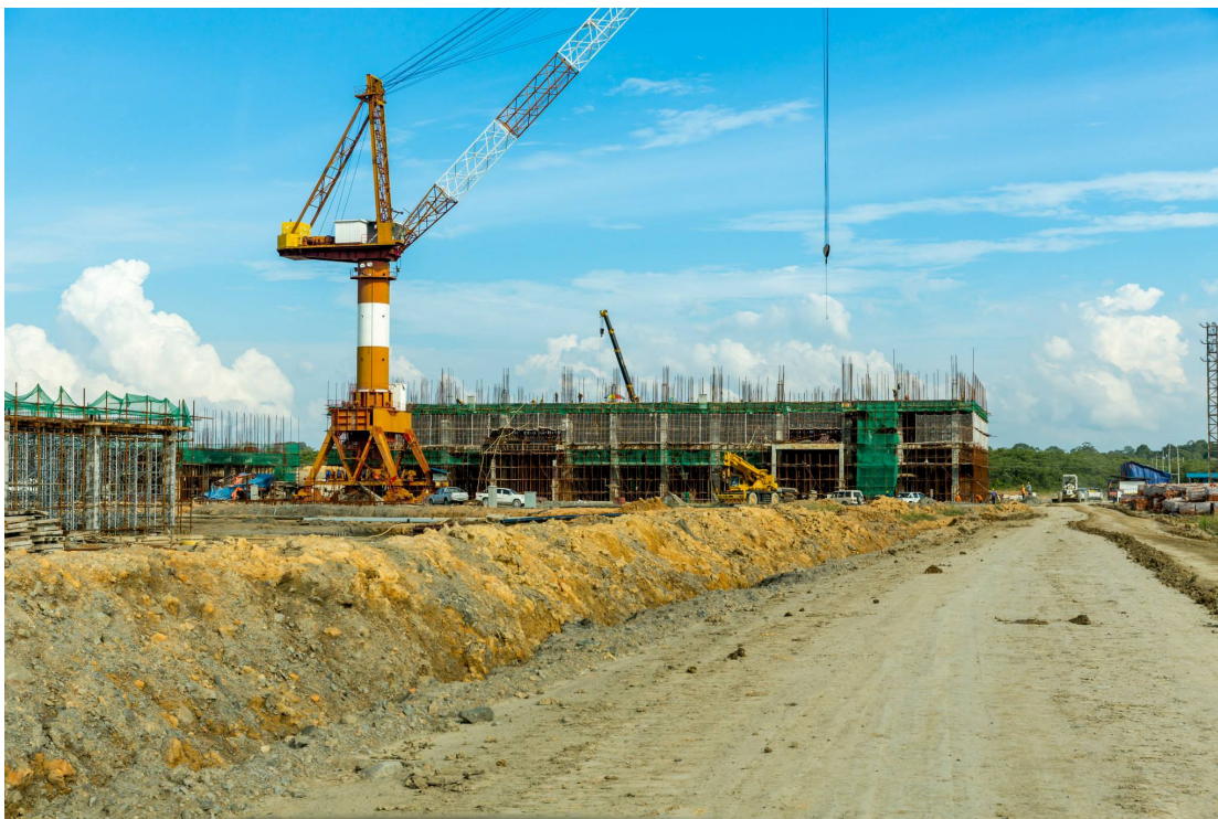
Main Furnace Building
