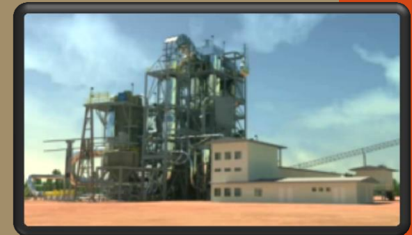
Briquette Processing Plant
