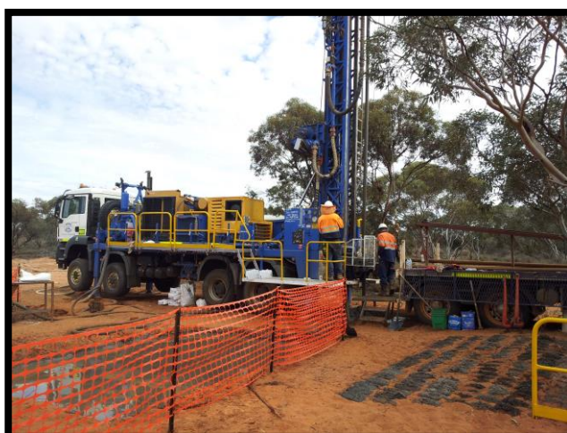
Bore field drilling commences at Hawsons
