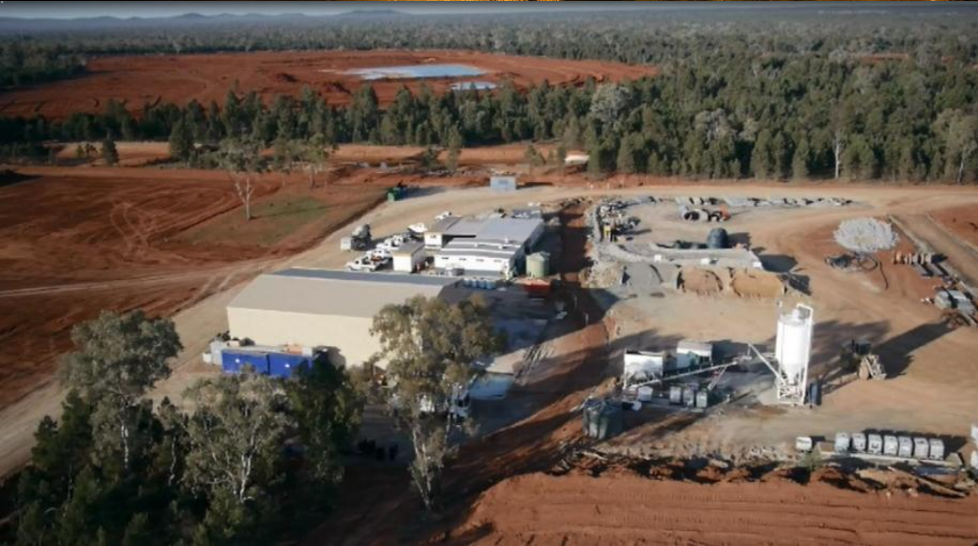
Hera Contractors area – looking south to TSF
