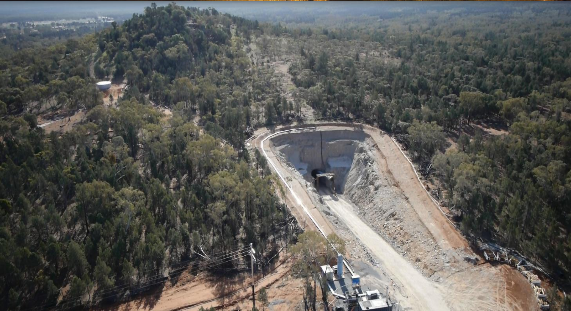
Hera Boxcut and Portal
