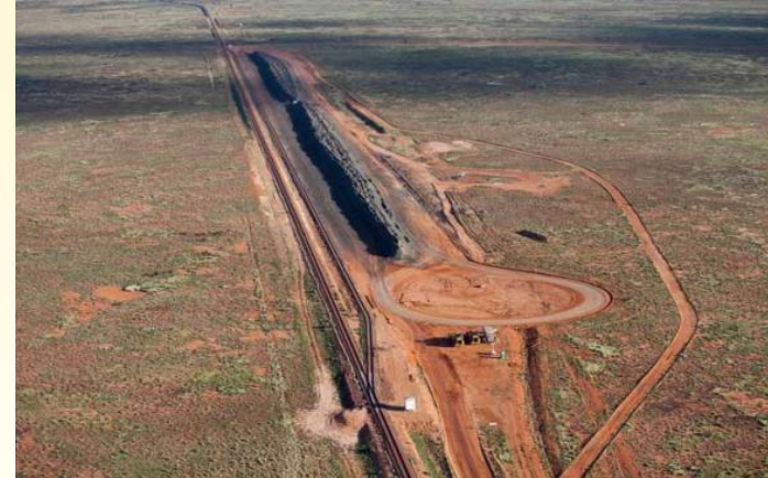
Rail Siding and Loading Facility
